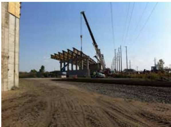
*Construction of a two-span steel bridge at Gary-Chicago International Airport. The new bridge spans over the EJ & E railroad tracks that bisect Airport Road near Chicago Avenue.*
