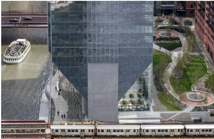
A multi-level green space connects 150 North Riverside and the parking structure immediately to greater Chicago in many different directions. Working with geofoam enables designers to create a custom contour of substrate material in the exact depth needed below specific planting areas. Photo: © Tom Rossiter Photography
