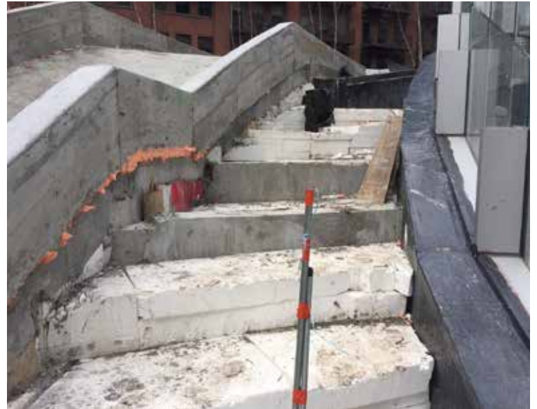
Lightweight geof foam blocks are easily maneuvered by two laborers and can be customized to virtually any shape with a hand-held hot wire cutter. Photo: ACH Foam Technologies
