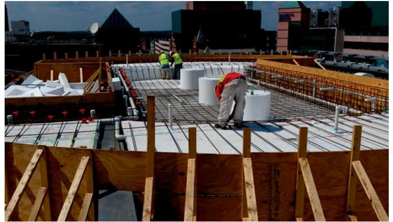
A rooftop pool is constructed on varying thicknesses of geofoam, ranging from 6 inches to 36 inches, to minimize the weight added to an existing parking structure.
