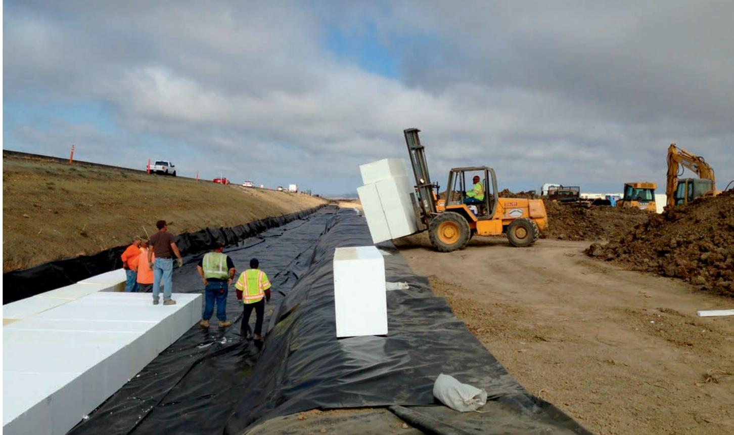
Geofoam wrapped with a gasoline-resistant membrane was placed in a new embankment slope along a Northern California highway to prevent roadway settlement during adjacent wetlands restoration..
