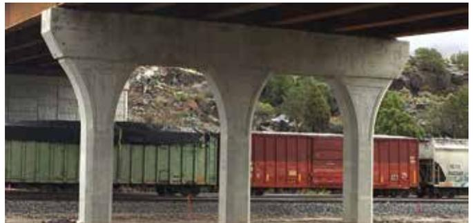
A completed pier, with three flared columns and pier cap, for the main bridge for the Cheyenne South Valley Connector in Pocatello, ID
