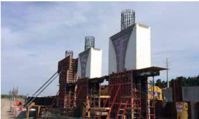
Cut foam blocks and fillets were delivered to the site, ready to be clamped into conventional wall formwork to form the three columns for a bridge pier. Here, the foam blocks have been exposed in preparation for installation of the pier cap formwork
