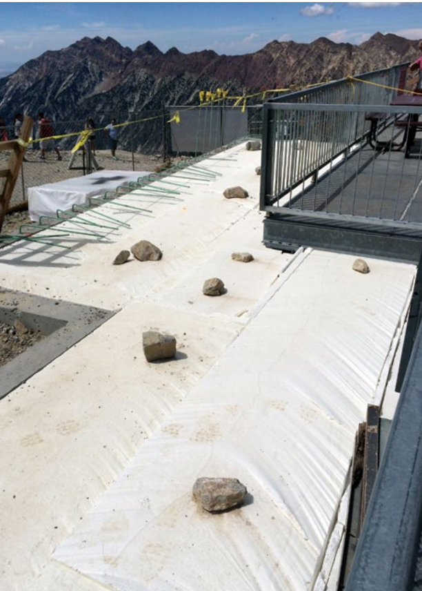
Installing geofabric at The Summit. Photograph courtesy of ACH Foam Technologies
