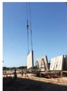
Enterprise uses a highly-specialized and proprietary wall system called the Altus CarbonCast panel which was developed by a conglomerate of architectural precast producers with exclusive ownership of the technology. Founded in 2003 under a “co-op-
